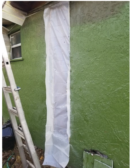
Figure 14. Unless you are a licensed and insured contractor, you should not attempt to repair a structure yourself. Flexible plastic sheeting can be used to provide a temporary seal. Credits: Jason Deeringer, Bee Serious Bee Removal, LLC
